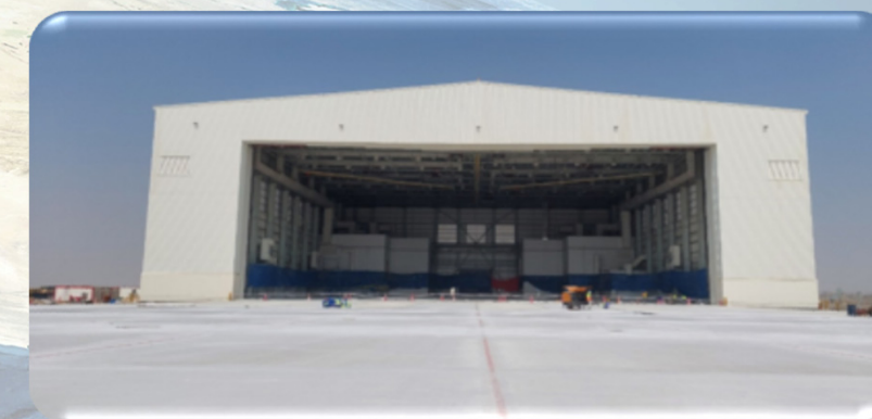
Large Aircraft Maintenance Facility, UAE Contractor: Amana Contracting & Steel Bldg WLL AE: Stanley Consultants
