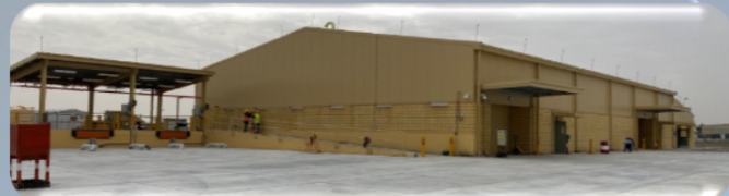
Super Hornet Warehouse, Kuwait Contractor: American International Contractors Inc AE: Adkins Global
