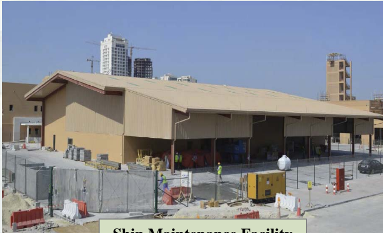
Ship Maintenance Facility
