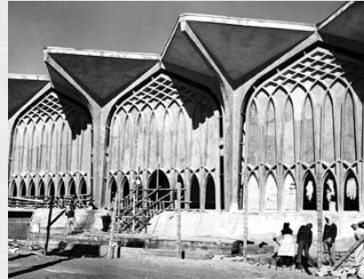
South face of the Dhahran Civil Air Terminal under construction, January 1961
